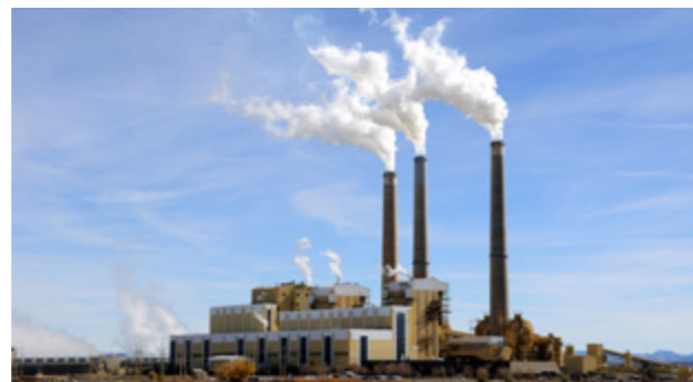
Longview Power Plant United States
