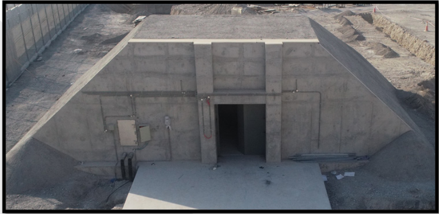
Picture: Typical Igloo Construction
